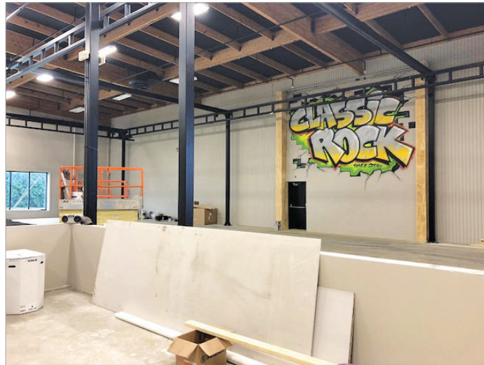
Classic Rock Fabrication, based in Lower Paxton Township, Dauphin County, is opening a design center in Mechanicsburg, as seen here. PHOTO/SUBMITTED
